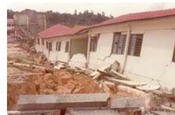
Figure 5: Slope failure due to rapid draw-down.
