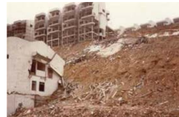
Figure 6: Slope failure associated with housing project in hilly terrain, KL.
