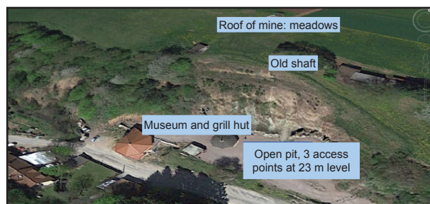
Figure 1: Satellite picture of the front cliff of the mine. The current rock front is a cleaned-up open cast mine, which is open for visitors during summer. The mine is run by an association, the Kupfermine Wilhelmine Sommerkahl e.V. The mine also hosts a small grill hut and a museum, which contains a rich collection of local minerals, and ancient mining tools.
