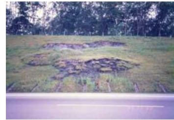
Figure 3: Slope failure in graphitic schist soils, Air Keroh.
