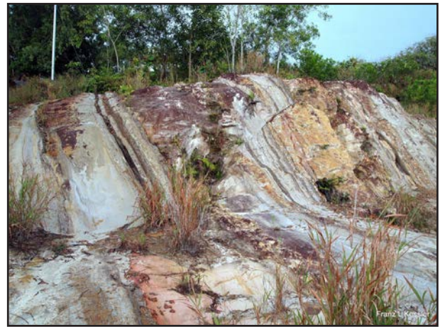
Figure 5: Kampung Lopeng Outcrop. Faulted and thrust sediments of the Tukai Formation are exposed, an excellent location for investigation of fault geometries and mechanics. Approximately face of outcrop height is 4m.
