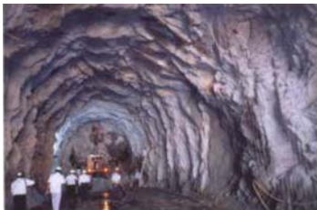
Figure 4: Diversion tunnel in granite, Sg. Selangor.
