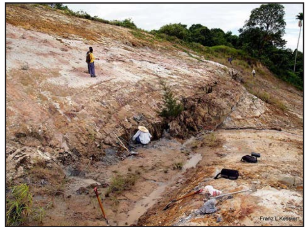
Figure 4: Oil seep location on the Canada Hill slope and above a Petronas gas station opposite the Meritz Hotel with observing geologists for scale.
