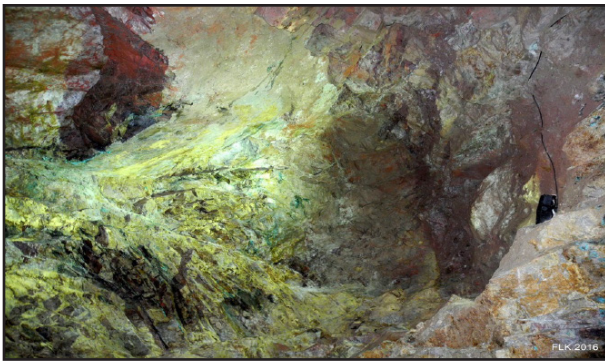
Figure 11: The Wihelmine mine. Due to very stable rock, no additional support is required.
