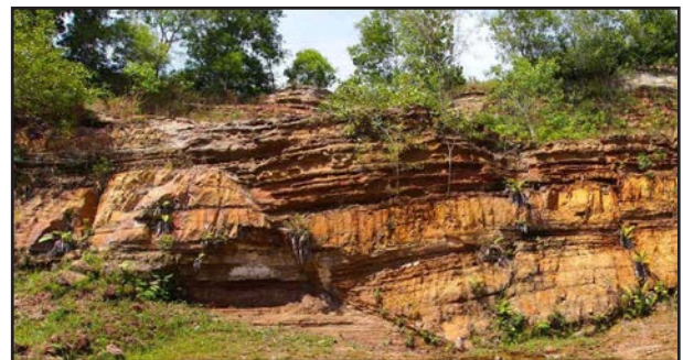
Figure 2: Miri Airport Road Outcrop. The main fault is interpreted as part of a crestal collapse structure of an inversion anticline, which forms the Miri Field. Approximately face of outcrop height is 6m. From Nichols & Baker, 2015.
