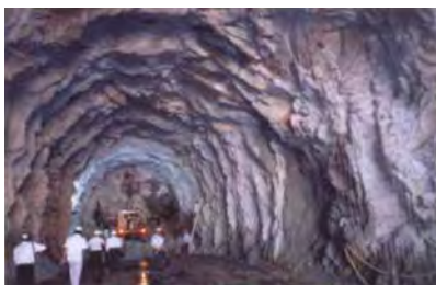
Figure 4: Diversion tunnel in granite, Sg. Selangor Dam.
