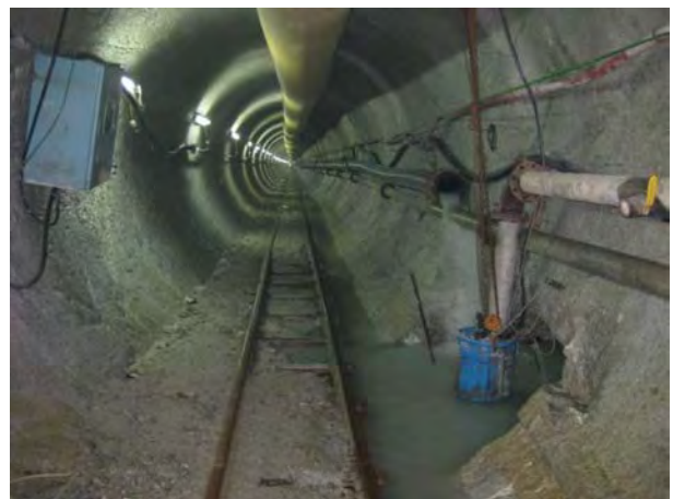
Figure 2: Smooth circular section produced by TBM in granite.
