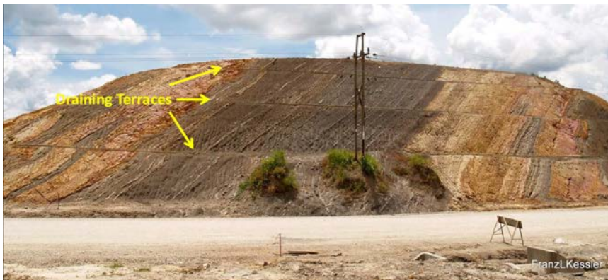
Figure 8: Outcrop section from the lowest part of Lambir Formation. Drains give the impression of faulting, which is an optical illusion. The sands appear mostly laminar-layered, are clean of shale, as well as of coal.
