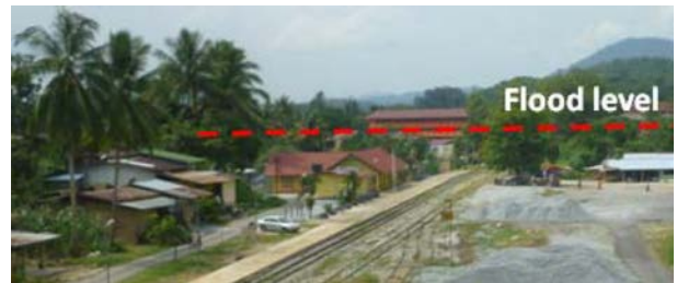
Figure 5: Flood level at Dabong train station.
