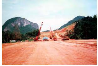
**Figure1:** North-South Highway under construction, looking north. G. Tempurung (limestone) on the left, schist in cut-slope on the right, and granite further right (Main Range). Colluvium occurs along the Highway mainly as valley fills.
