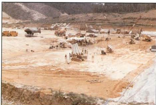
Fig. 14. Foundation grouting at Batu Dam, K.L.
