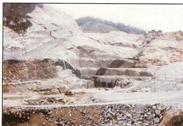
Fig. 15. Kenyir Dam, a rockfill dam, Kuala Berang, Terengganu. Dolerite dykes (black) in granite.
