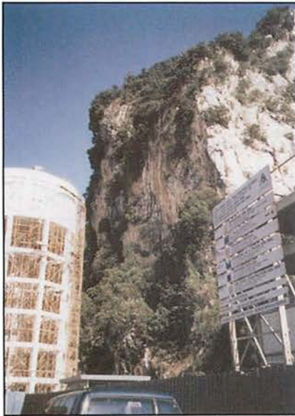
Fig. 4. Water tank at Batu Caves limestone cliff, Kuala Lumpur.
