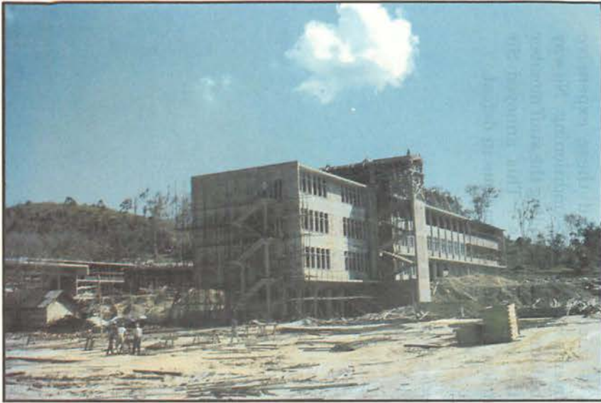
Figure 8. Chemistry Department under construction.
