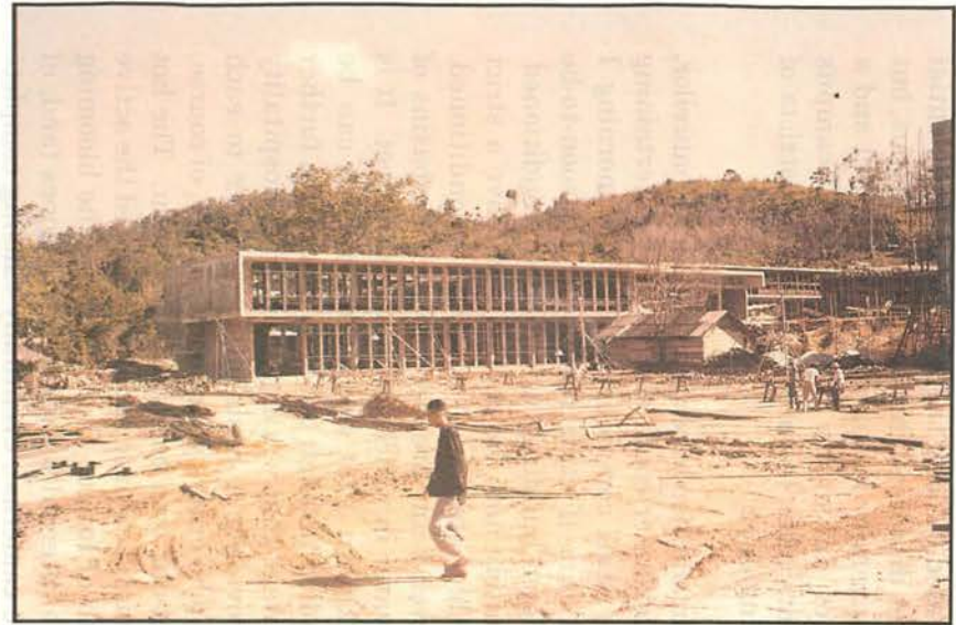
Figure 9. First Geology/Mathematics Department under construction.
