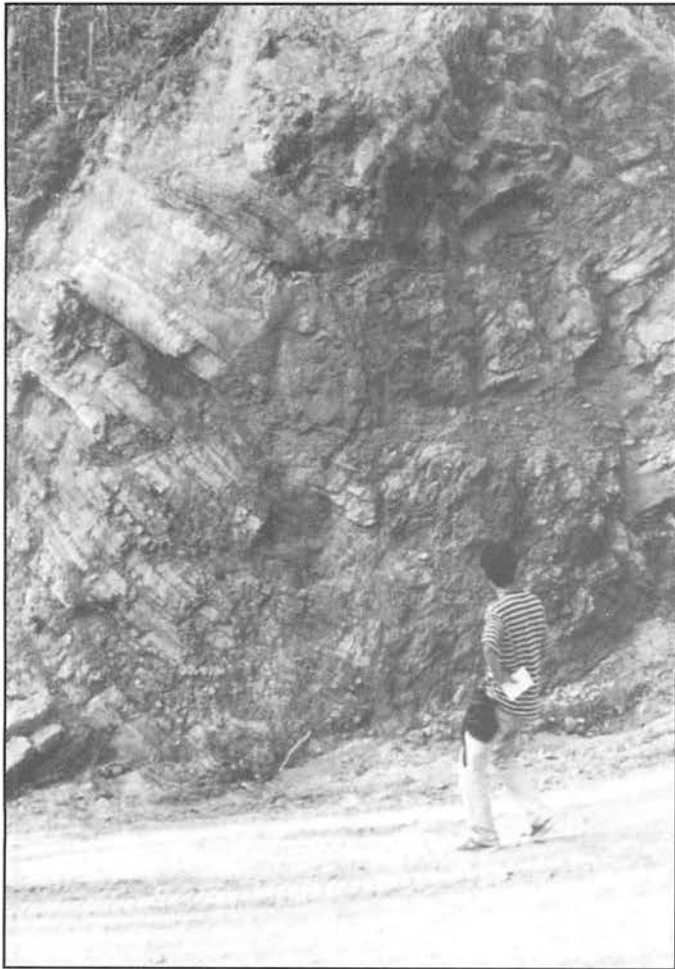
Figure 2a. The Tubau Fault zone in the Ulu Suai Dome. View is towards south parallel to fault strike.
