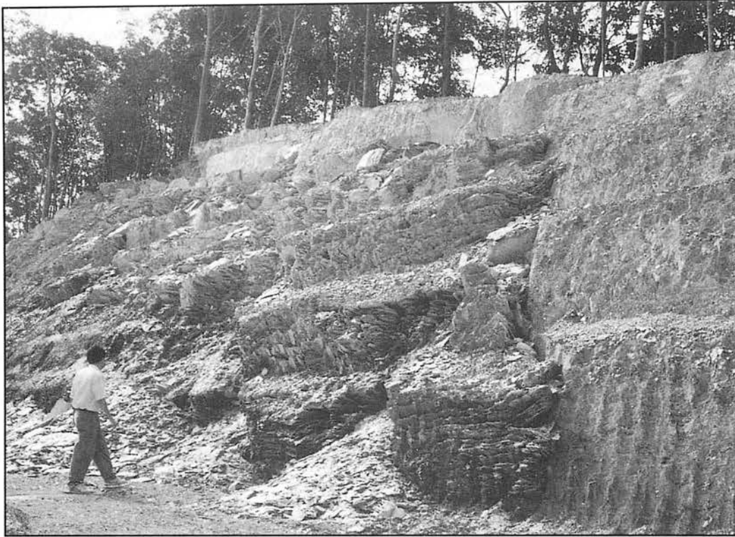
Figure 5. CH9300L. Fault ( f_1 = 328/90 ) on right side of slope along which failure has occurred.
