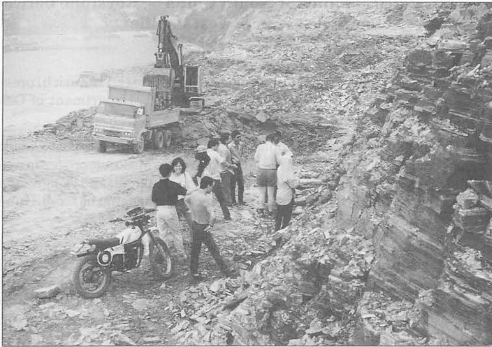
Discussion at Batu Arang quarry. Thrust fault or coal seam split ?
