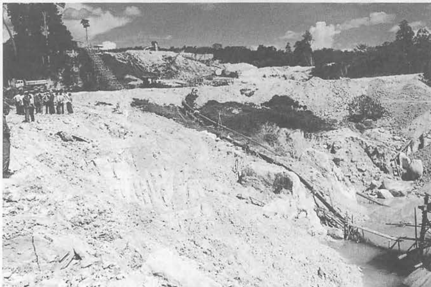
At the new mine pit at Sejati Jadi, Kechor Tui
