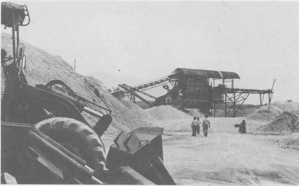
Plate 4. Crushing plant and stockpiles of rock aggregates.
